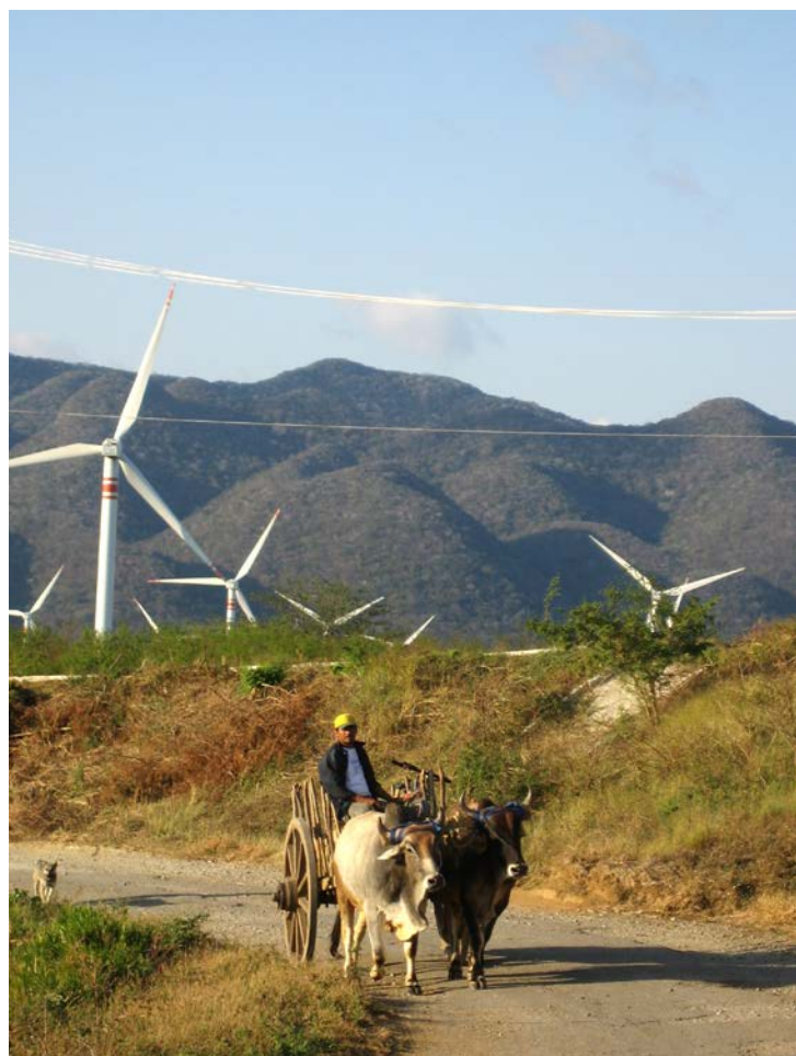
Oaxaca wind farm in Mexico.
