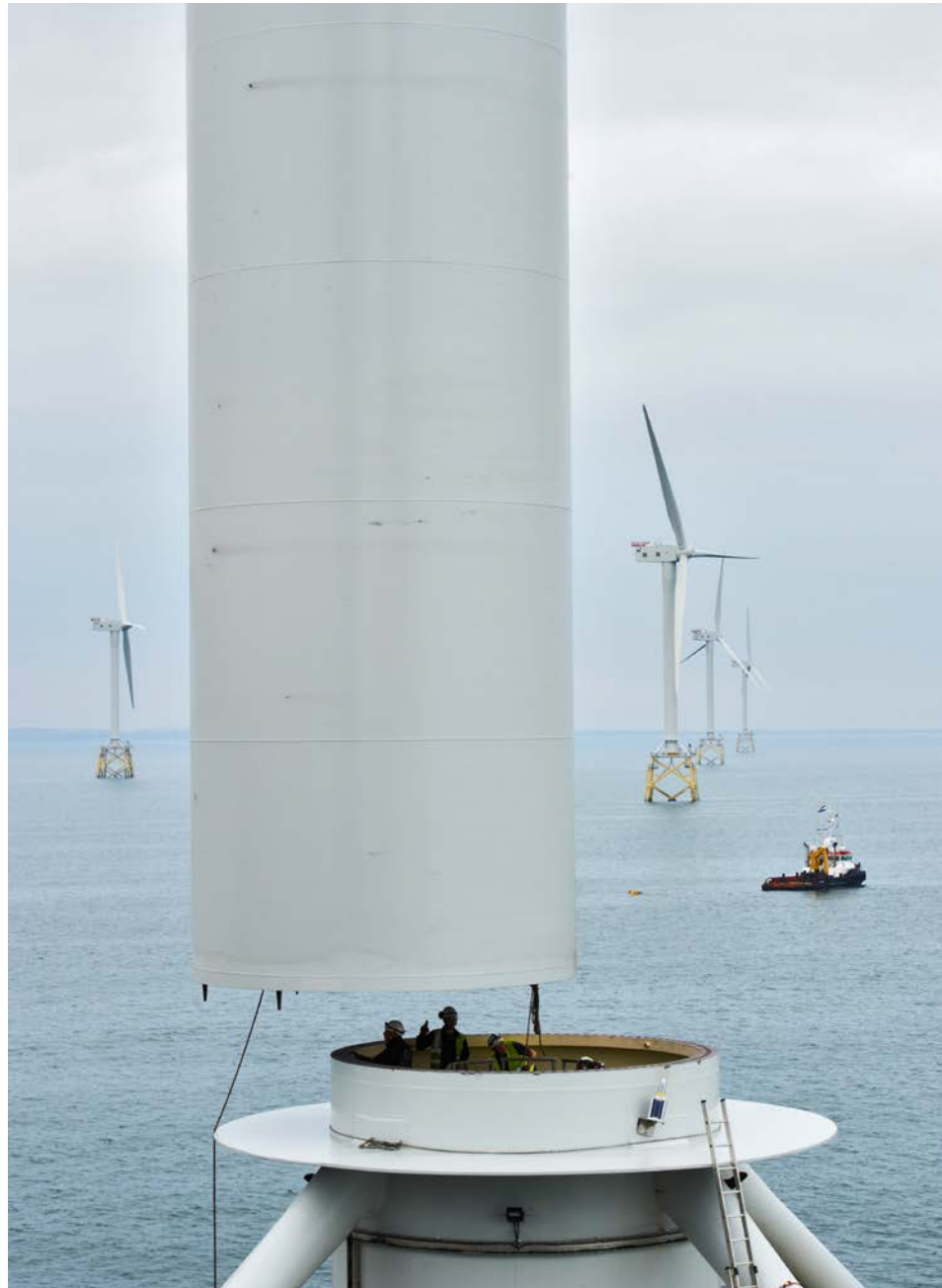
Construction of Ormonde offshore wind farm in the Irish Sea.
