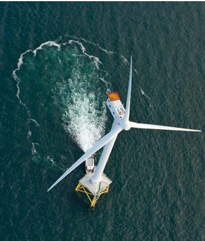
Repower-turbine in "Ormonde" offshore wind farm, UK.
